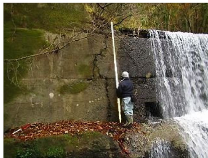
堰堤亀裂
